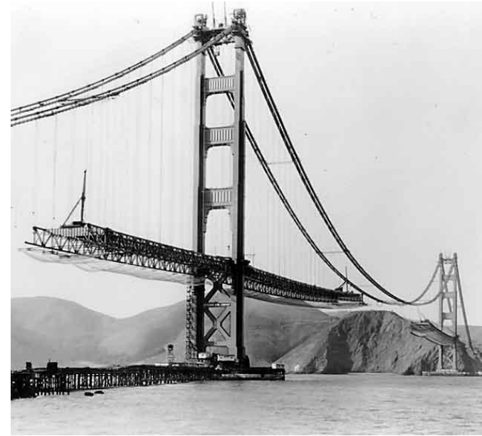
Golden Gate Bridge
